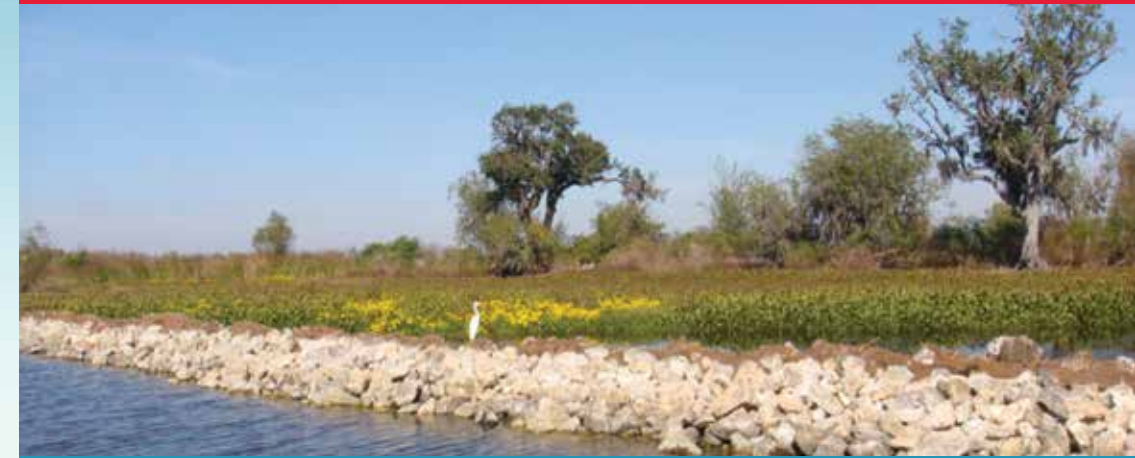
The Bayou Segnette cypress reforestation project in the Barataria Preserve included construction of protective rock jetties to reduce erosion.
